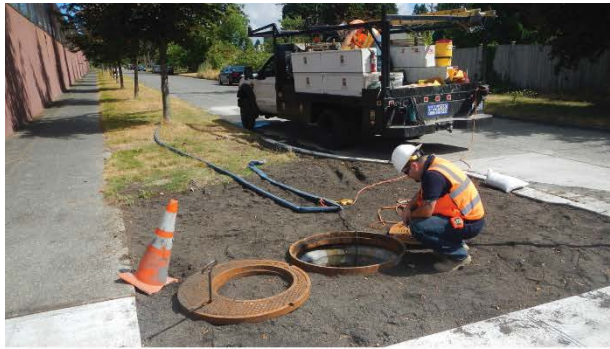
UMH easily accessed away from bioretention. Preferred.
