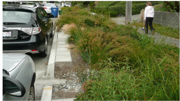
Tight pavers step out zone after installation
