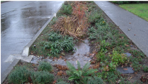
Facility with graded side slopes during storm event. Notice winter conditions may compromise the space in the step out zone
