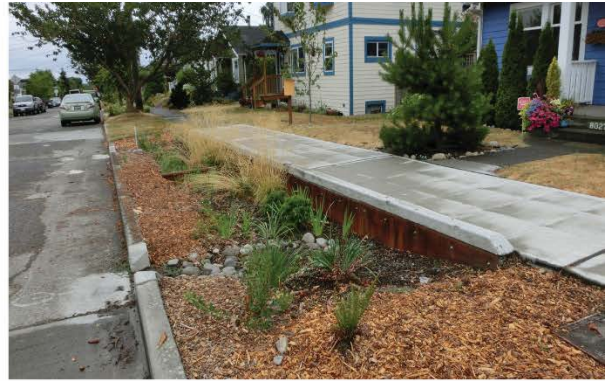
Bioretention with 1-sided wall and remaining sides sloped. Requires special review for wall design. Wall shall extend 18" beyond top of slope.
