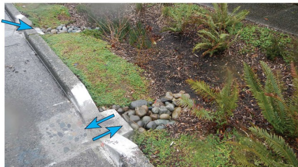
Drain curb cuts meets COS Std. Plans 295b and 295c.
