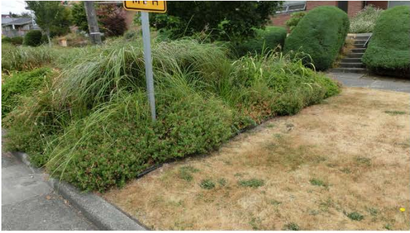
Landscape edging defines end of facility
