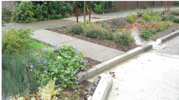
Pervious concrete access path
