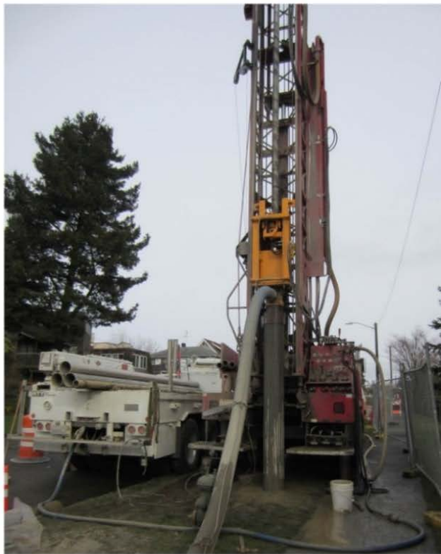
Larger rig used to drill UIC wells
