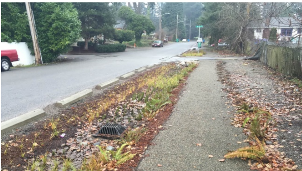
Gap curb rain garden facility, notice leaf accumulation is addressed by inlet, 32nd Ave NE, Shoreline
