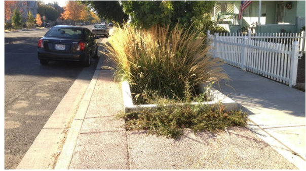
Concrete step out zone and access path
