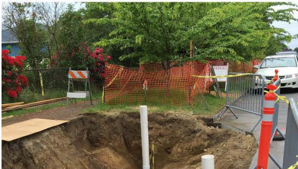
Existing street tree protection
