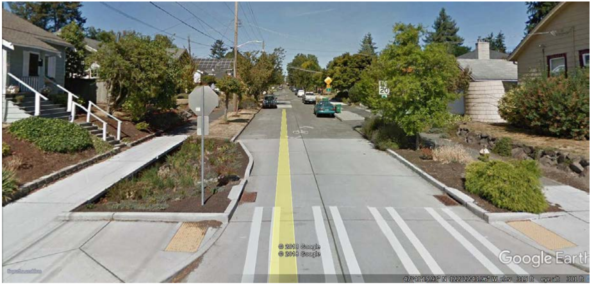
Image: Bioretention with vertical wall at sidewalk in new curb bulb just after construction. Less than 2-foot setback provided from edge of ramp to top slope of bioretention cell.
