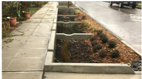
Review need for weirs and provide wider intervals
