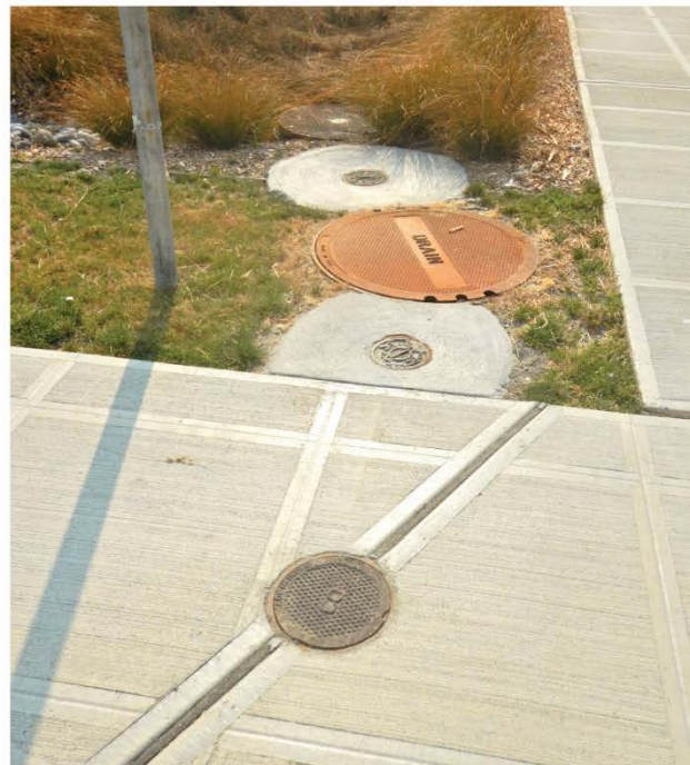
Valves that require concrete collars should be placed in sidewalk or review location to minimize impact.
