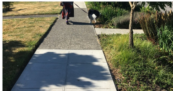
Existing sunken sidewalk was replaced as part of construction of bioretention cell in planting strip.
