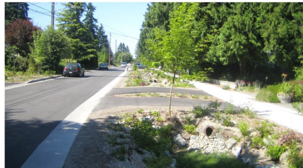
Curbless facility, avoid steep side slope, Broadview Green Grid, Seattle
