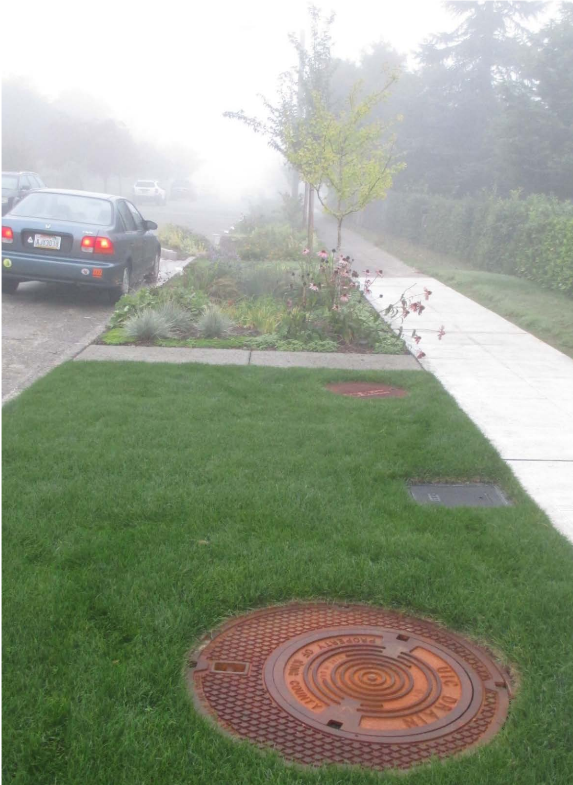
Image: Dual opening UIC screen well lid (foreground) and underdrain MH access lid (background) located downstream of bioretention cells on a Neighborhood Yield street.
