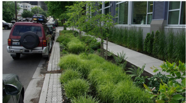
Paver step out zone - difficult to weed
