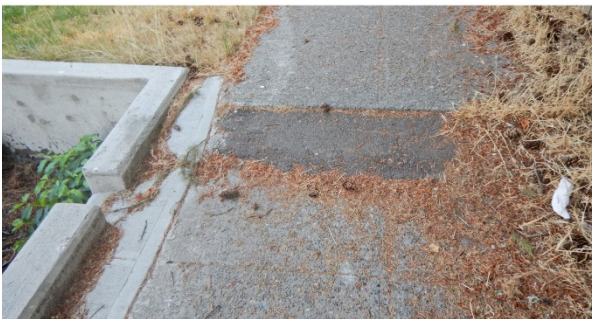
Recommend sidewalk replacement when a section is uplifted next to a new facility. Sidewalks adjacent to cell with vertical wall are to be replaced.
