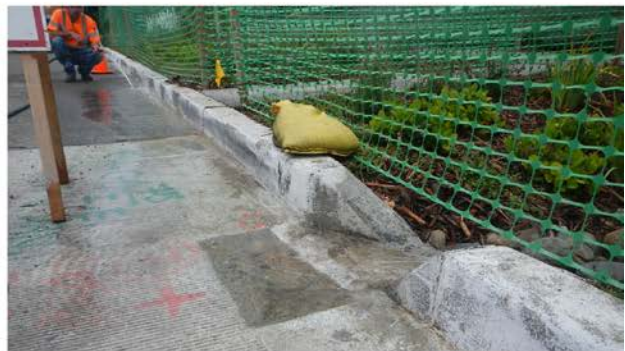
Gutter flow testing during construction
