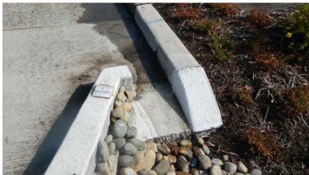
Gutter flow testing during construction
