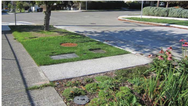
MH and irrigation boxes located outside of bioretention cells in lawn area for easy access.
