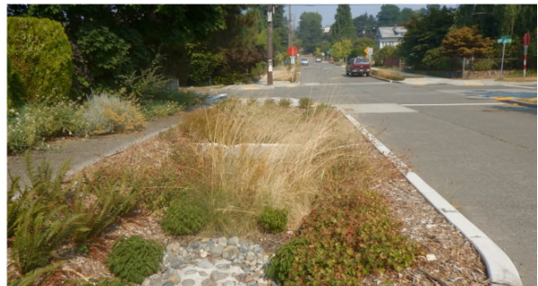
Curb bulb with bioretention with graded side slopes, concrete weir and presettling concrete pad. Notice plants held back to allow for clearance at step out zone along curb
