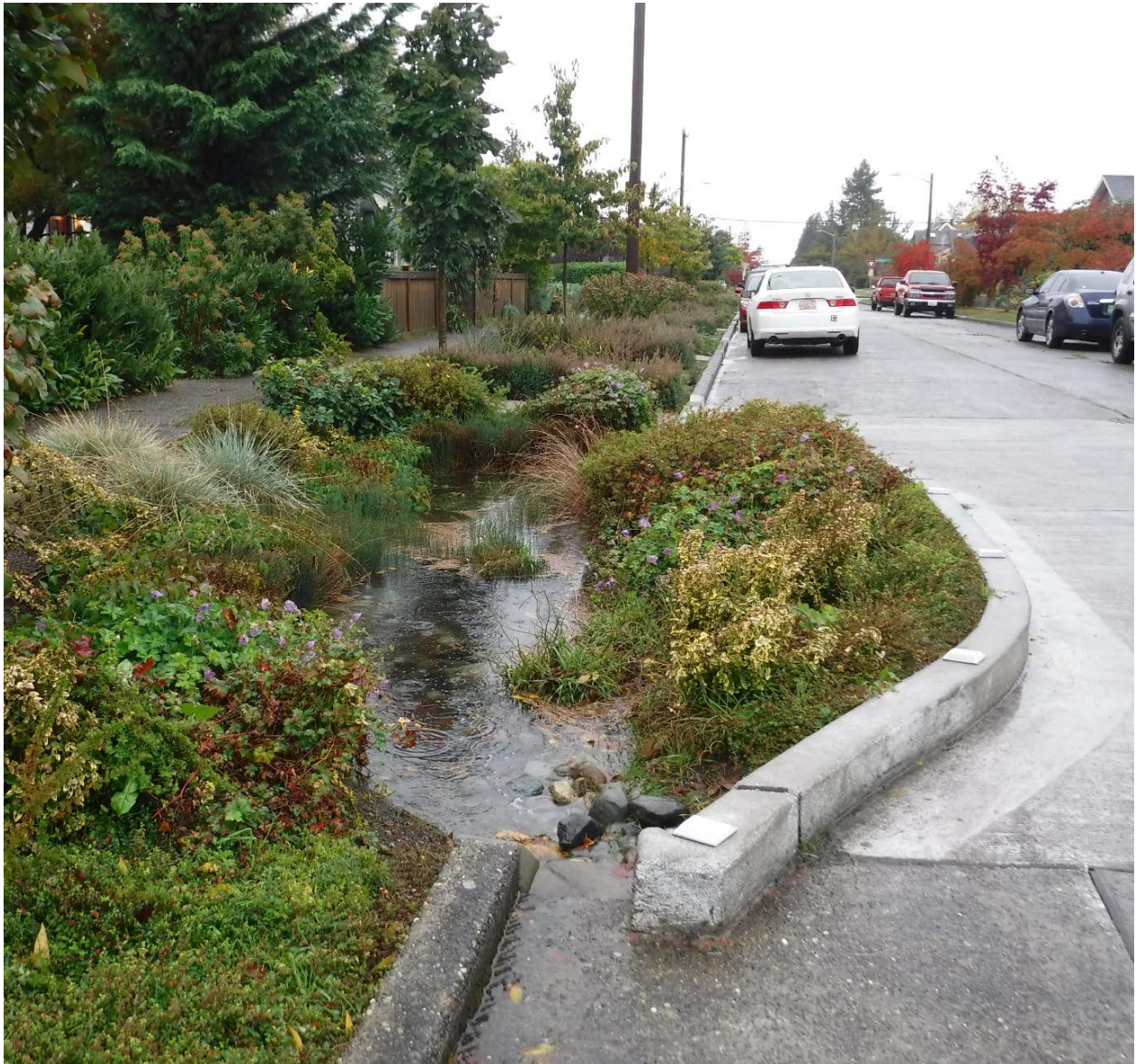
Image: Bioretention cell with curb bulb constructed for WTD's Barton CSO Control with GSI project in West Seattle.
