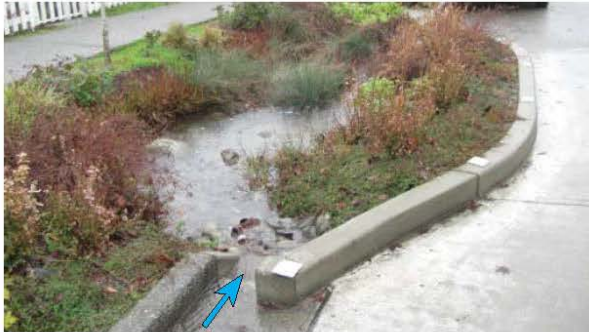
Presettling cell during rain event, meets COS Std. Plan 295d
