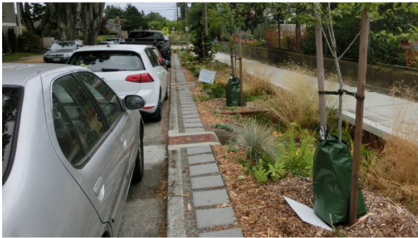
Paver &amp; gravel step out zone
