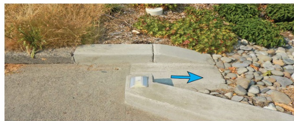
Drain curb cut does not meet COS Std. Plan 295d. Missing vertical drop from gutter to top of bay.
