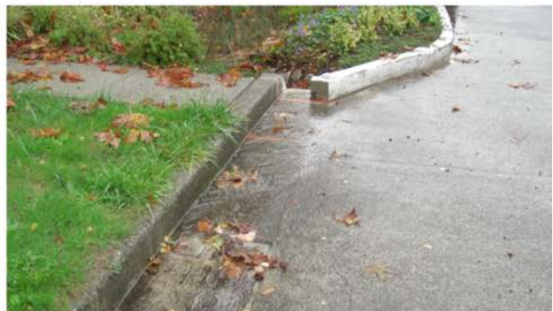
Street gutter flow into curb bulb drain curb cut
