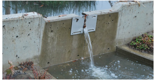
Weir aperture blocked by debris. Requires special review. Weir slot too small for practical ability to keep open
