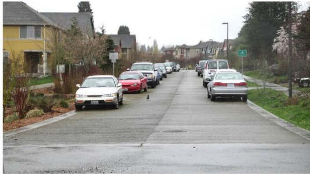
Pervious concrete curbless street
