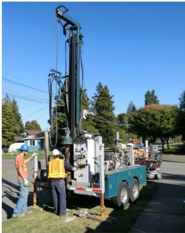
Smaller rig used to drill monitoring wells
