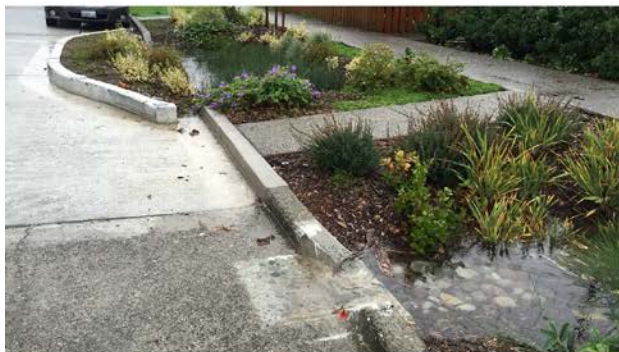
Street gutter flow into drain curb cut
