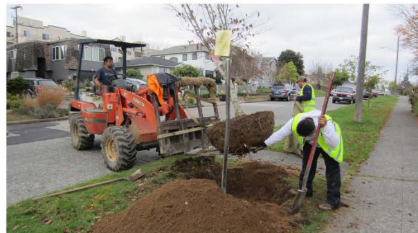
Transplanted existing street tree
