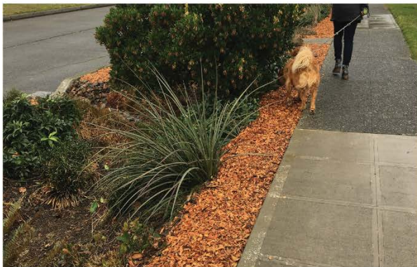
Bioretention with sloped sides on Neighborhood Yield, COS Std. Plan 293a. Fourth winter season.
