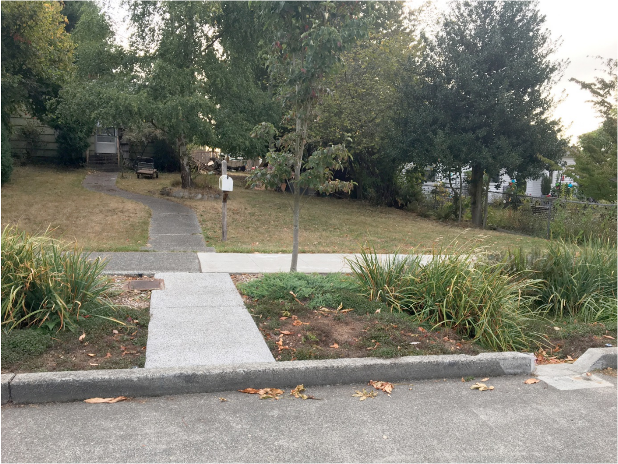
Image: Pervious concrete path and new street tree in level area between bioretention cells with graded side slopes on Neighborhood Yield street.
