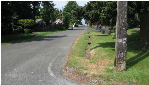
Existing ditch conveyance
