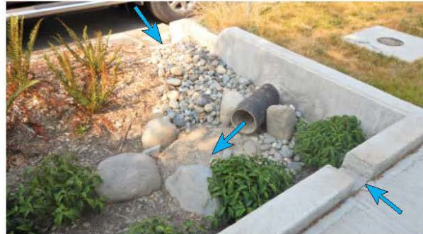
Cobbles at pipe discharge point. Presettling pad per modified COS Std. Plan 299
