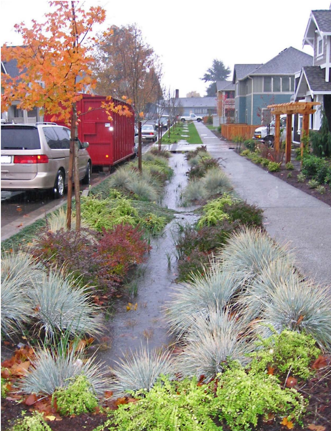
Image: A series of bioretention cells (vegetated and grass lined) along a new Neighborhood Yield street in High Point neighborhood during heavy rainfall event on November 6, 2006.
