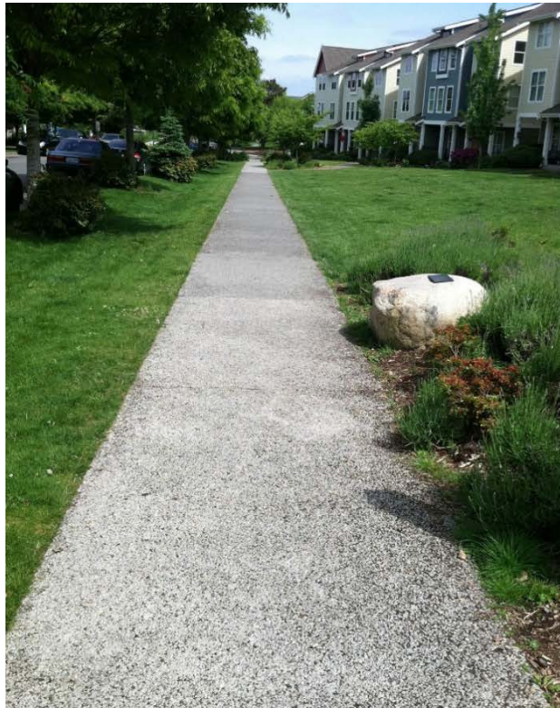
Pervious concrete sidewalk
