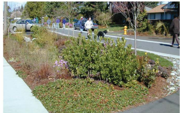
Bioretention with sloped sides on Neighborhood Curbless, COS Std Plan 292.
