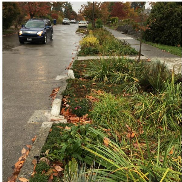
Facility with graded side slopes during storm event. Notice winter conditions may compromise the space in the step out zone
