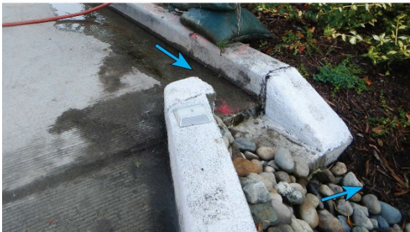
Drain curb cut meets COS Std. Plan 295d.
