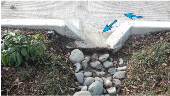
Primary drain curb cut meets COS Std. Plan 295b.
