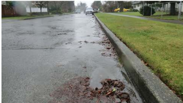
Gutter flow review
