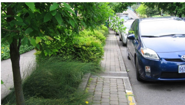
Paver step out zone - difficult to weed
