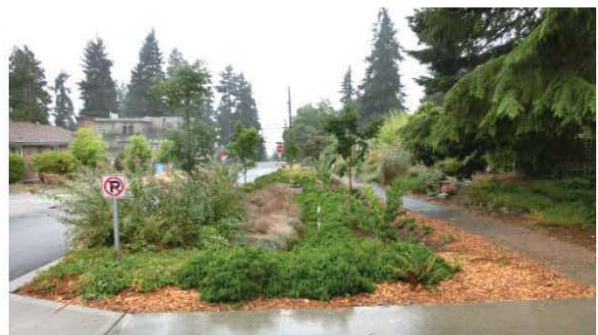
Plant availability: substitution blocks alley sight lines
