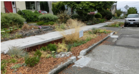
Bioretention facility with one vertical wall. Notice abrupt change of condition along the block
