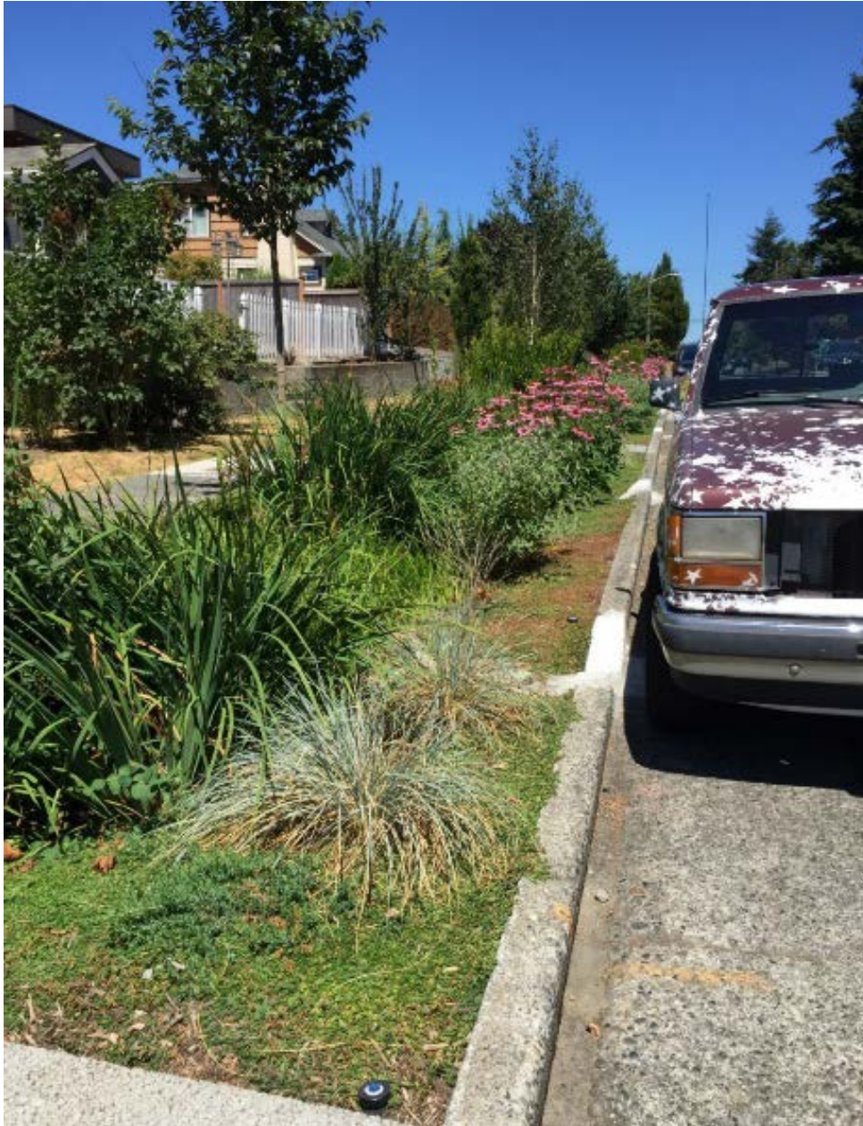
Image: Basic retrofit of planting strip with bioretention cell for WTD's Barton CSS basin for CSO control in West Seattle.
