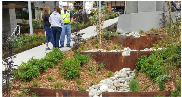
Corten steel weirs example. Recommended top edge, especially sidewalk edge, be treated (such as round molding) to avoid sharp edges
