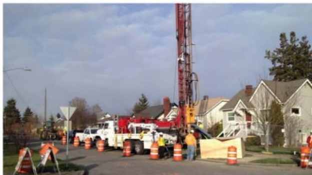
Larger rig used to drill UIC wells
