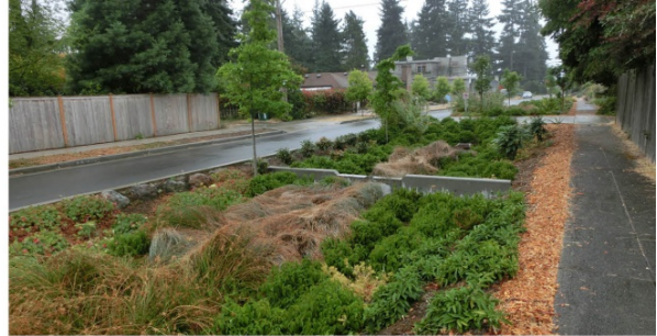
Wide bioretention facility with weirs. Full ROW retrofit managing flow from multiple blocks. Recommend allowing more space along sidewalk so as to not constrain pedestrians with steep slope of cell and fence at walk.
